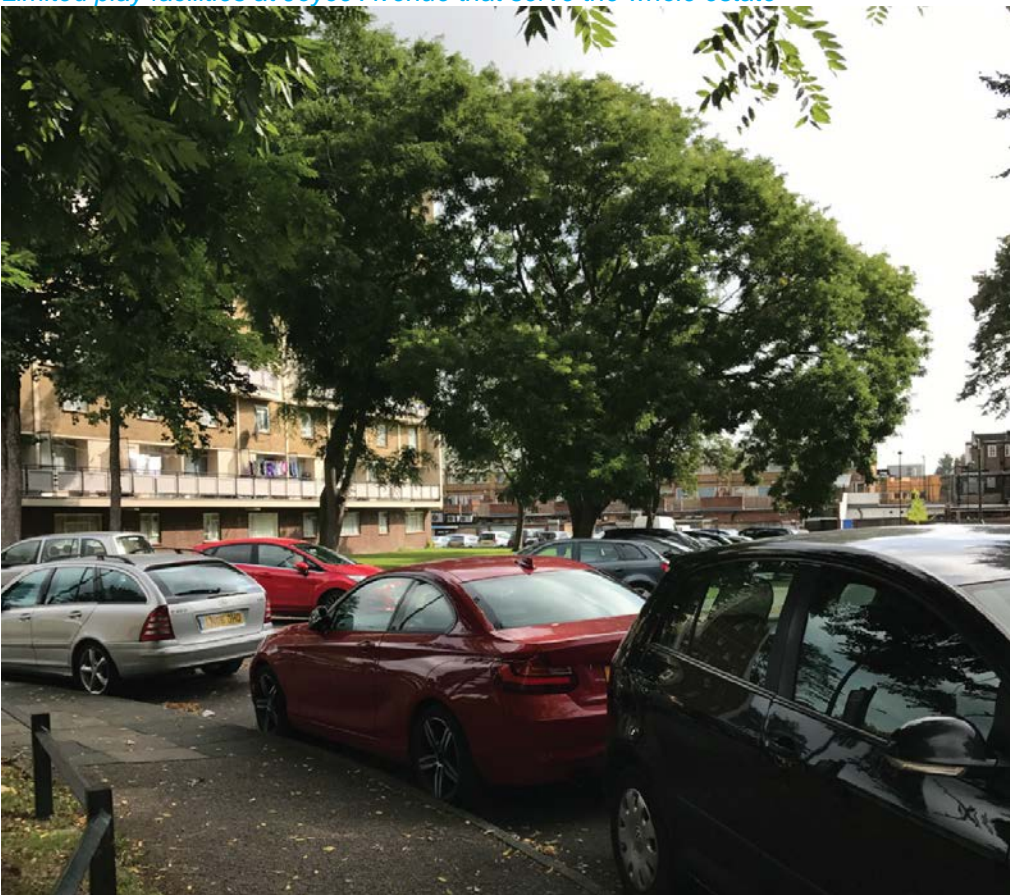
The estate is heavily parked with residents and commuters. CPZ only operational on match days. The estate was designed at a time of much lower car ownership. Parking impedes service and emergency vehicles
