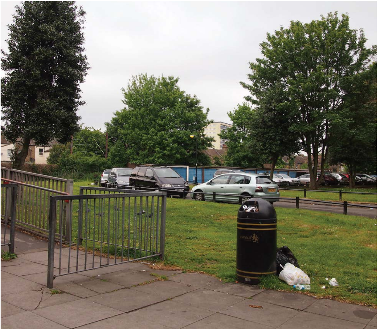
Entrance to estate over railway footbridge from the west, heavily used by hospital patients and visitors accessing the high street, as well as local residents. Undefined open ground, lack of overlooking and underused garage areas are spaces where ASB and crime can take place. Littering is problematic across the estate and in the High Street
