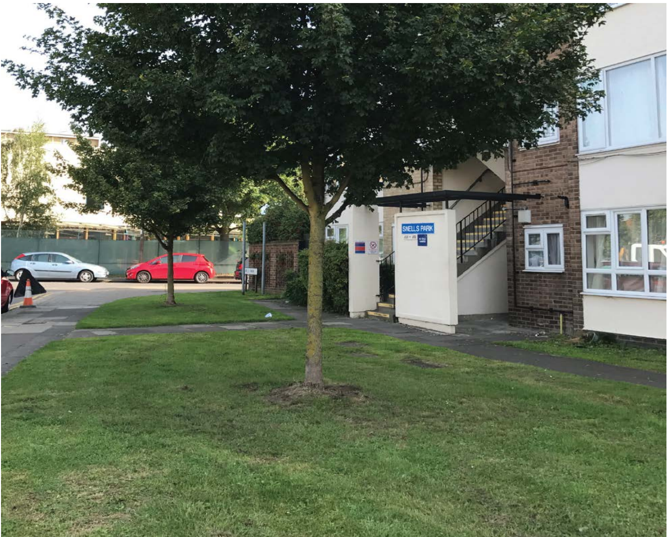
Open access stairwells and no defensive space around ground floor homes enable crime and ASB to take place
