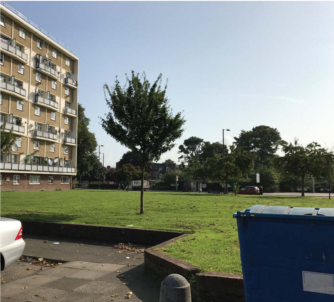
Open space with low ecological value. Bins stored externally across the estate - bin stores out of use due to ASB
